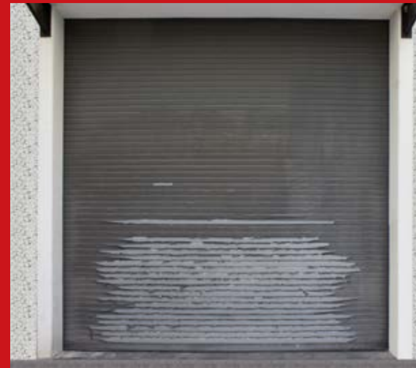
PVC coated steel shutter exposed to the elements
